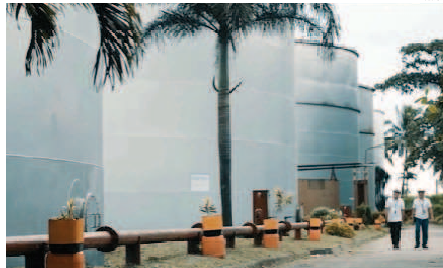
Waste Water Reactors at Distileria Bago, Inc.
